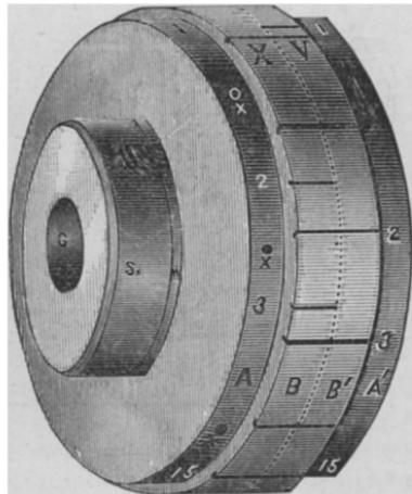
FIG. 2.—Drum of the new micrometer-screw.
