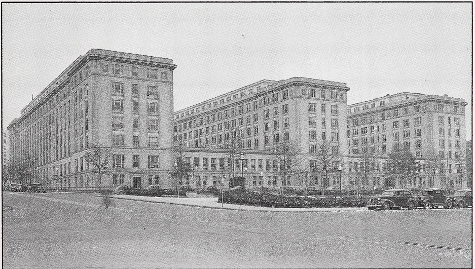
The Second Interior Building, 1917-1936
